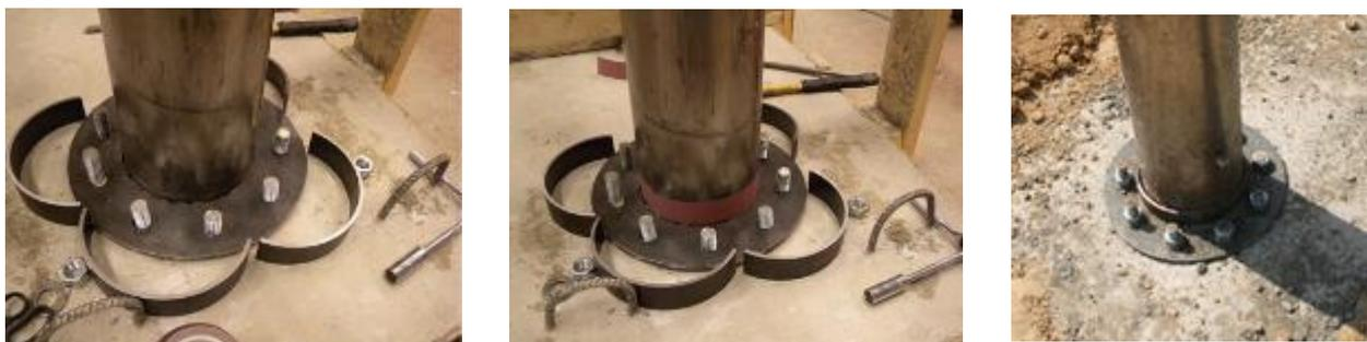
Figure 8. Steel Collar: Components (Left and Middle) and Construction (Right)
